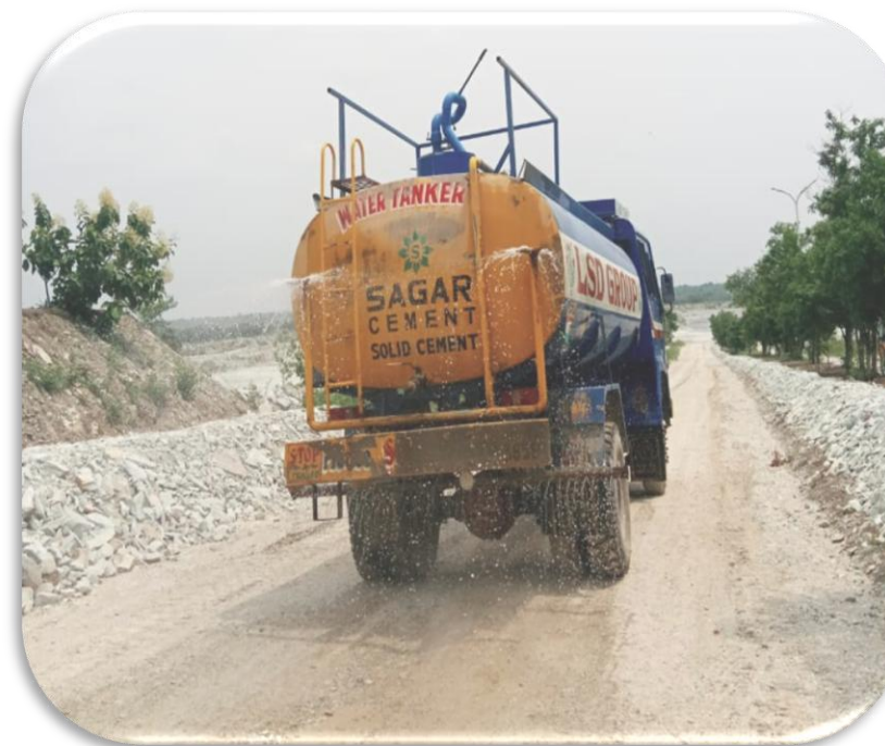
Water Sprinkling on Haul Roads & Muck pile wetting
